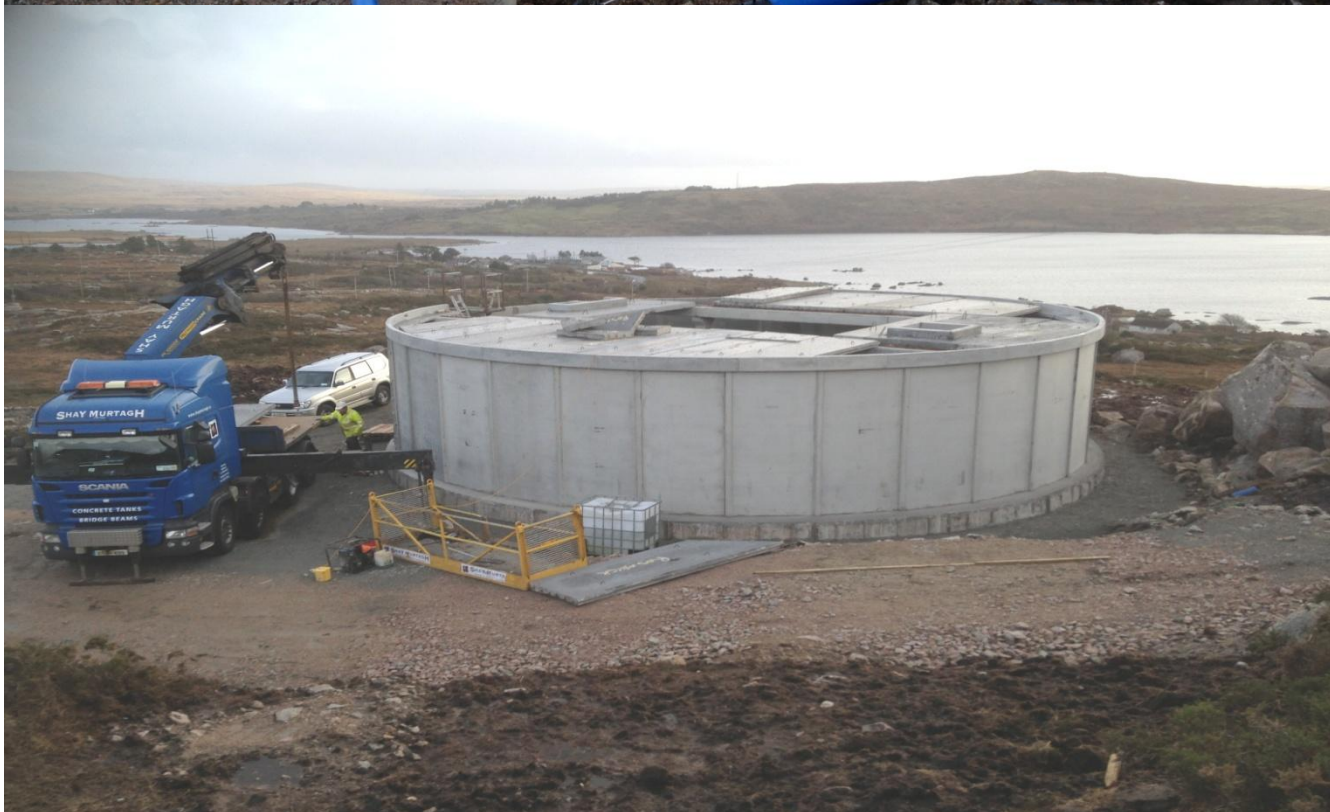
Pictures above show construction work at the 2 reservoirs in Costello
