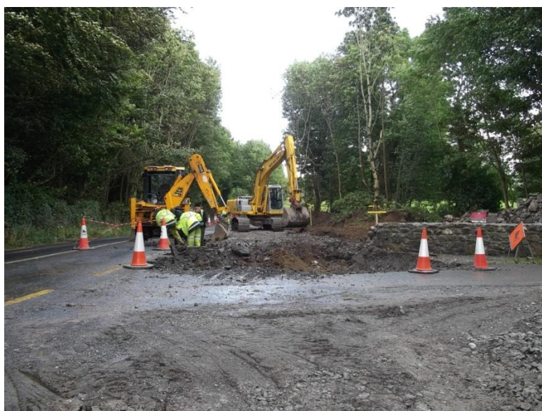
Roadworks in the Oranmore Area
