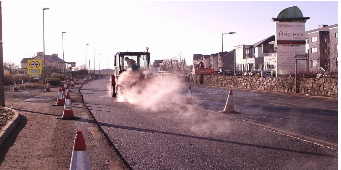
Pictures above show work in progress on the Milltown and Claregalway Sewerage Schemes.
